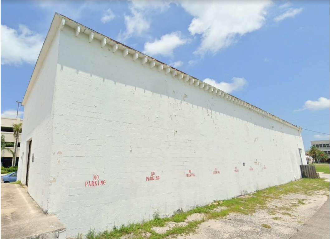
3. Commercial Building (east façade) – 701 Franklin Street
